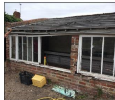
Image 6: Southern elevation showing the original timber windows which are damaged and in a very poor state of repair.
