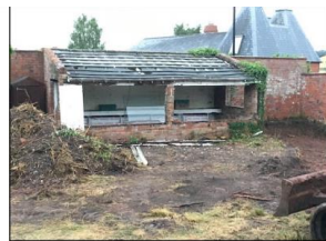
Image 6: Southern elevation showing the original timber windows which are damaged and in a very poor state of repair.
