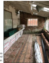
Image 5: Internal view of the Glass House showing Godwin floor tiles and deflection to the roof structure over.
