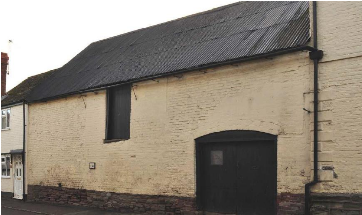
Figure 4: Subject barn prior to conversion showing an absence of openings to the roof slope
