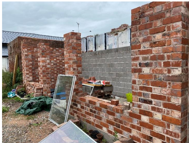
Site photo of partially reconstructed Glass House (July 2020)
